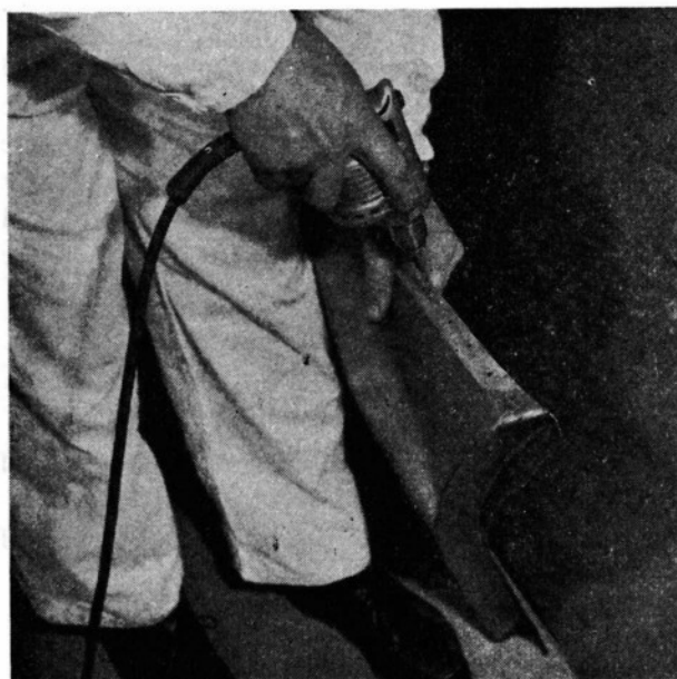
Drilling holes for plug welding
