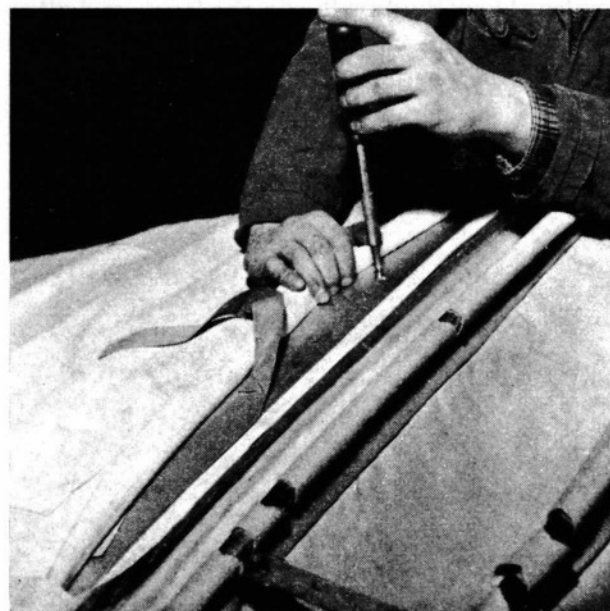
Attachment of outer fabric at rear edge.
