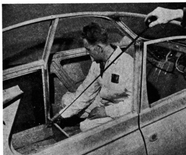
Diagonal measurement of center pillar location
